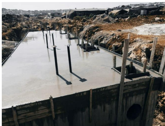
Figure 10: Constructed Septic Tank
