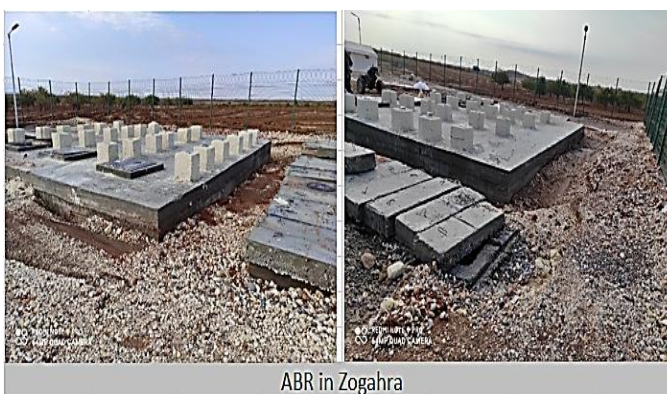
Figure 14: Anaerobic Baffle Reactor in Zoghara Camp Jarablus Aleppo Turkish Border
