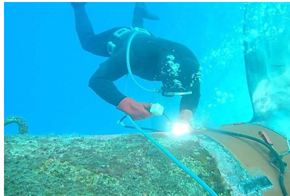
Figure 2: A Welding from Underwater
